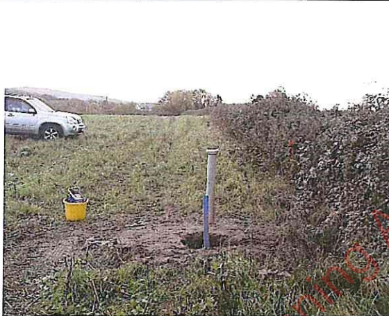
Photo 3 Piezometer Installation BH 1 pre-capping view towards south west (17/10/2018)
