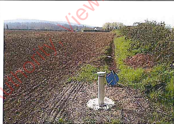
Photo 4 Piezometer Installation BH 1 completed view towards south west (10/4/2019)
